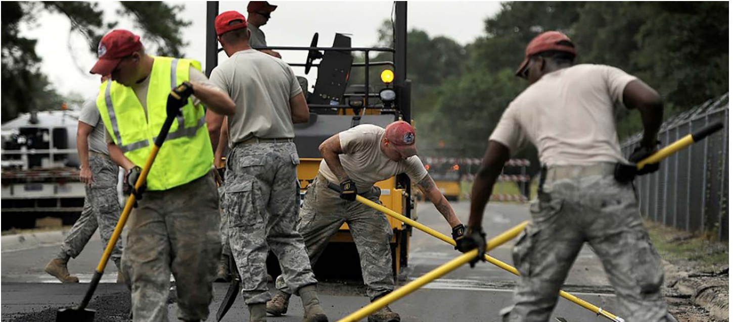
Interested in a skilled trade? Prepare now to be ready when Connecticut's highway and bridge projects break ground.
